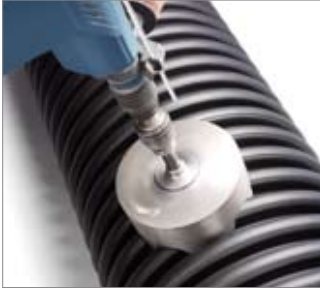
Step 1: Drill the borehole on main pipe
