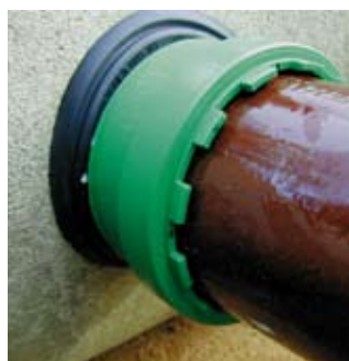
Clay to concrete pipes
