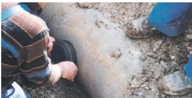
Screw the AWADOCK screw sleeve into the connecting seal
