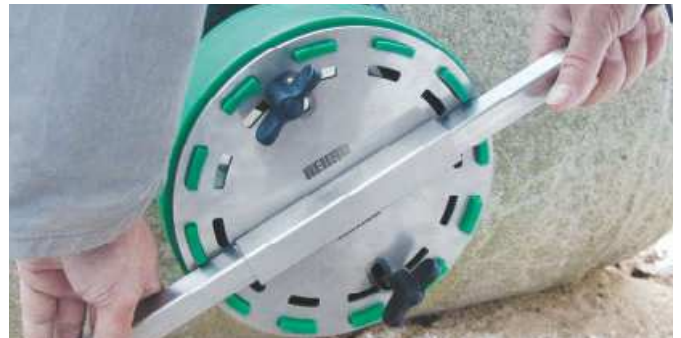
Insert the AWADOCK connecting seal into the hole
