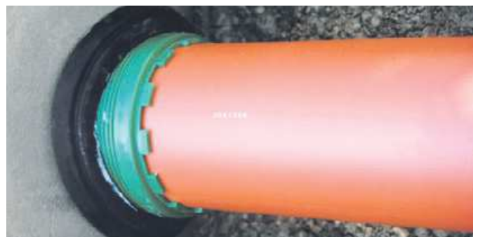
Insert the pipe into the AWADOCK screw sleeve up to the rebate
